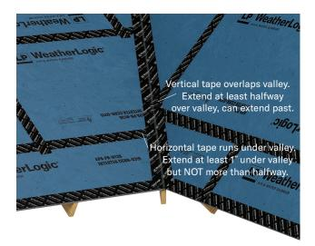
• 6"LP WeatherLogic® Seam & Flashing Tape is recommended. Center tape in the valley. Use the included squeegee to crease and tightly push the center of the tape fully into valley. Adhere tape to both sides of valley.
